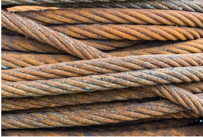
Slika 10: Korozirano čelično uže ( https://www.wire-rope-direct.com/wp-content/uploads/2016/10/Corroded-Wire-Rope.jpg )
