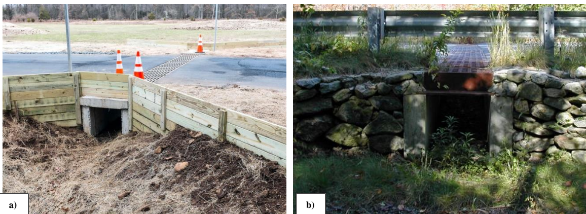
Slika 6.: a) Drvena ograda s propustom ( https://www.njfishandwildlife.com ), b) Kamena ograda s propustom ( https://climateactiontool.org )
