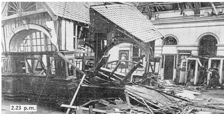
Sl.br.4 Izgled željezničke stanice York Road nakon eksplozije https://cain.ulster.ac.uk/events/bfriday/nio/photo7.gif 22.08.2021.
