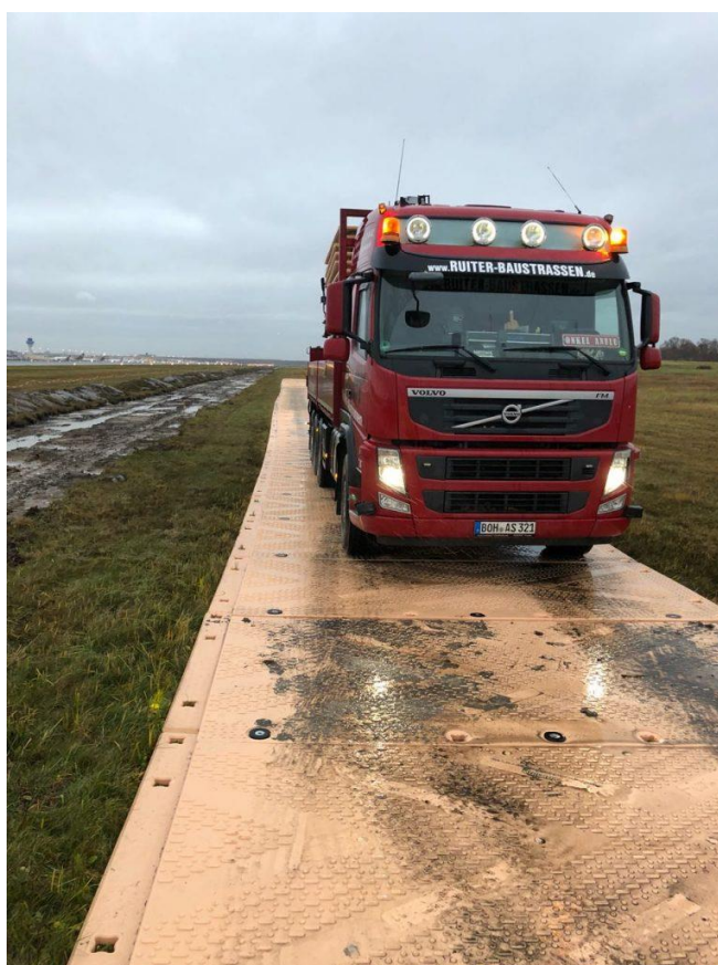
Slika 8. Transport kamiona po Isotrack X umjetnim podlogama ( https://www.isotrack.eu/images/pdf/Isotrack-L-brochure.pdf )
