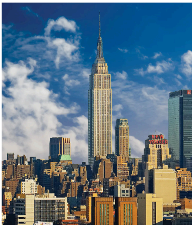
Slika 2. Empire state building [2]
